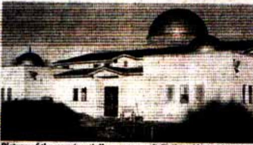
Picture of the new (partially constructed) Ba'itun Nasir Mosque
